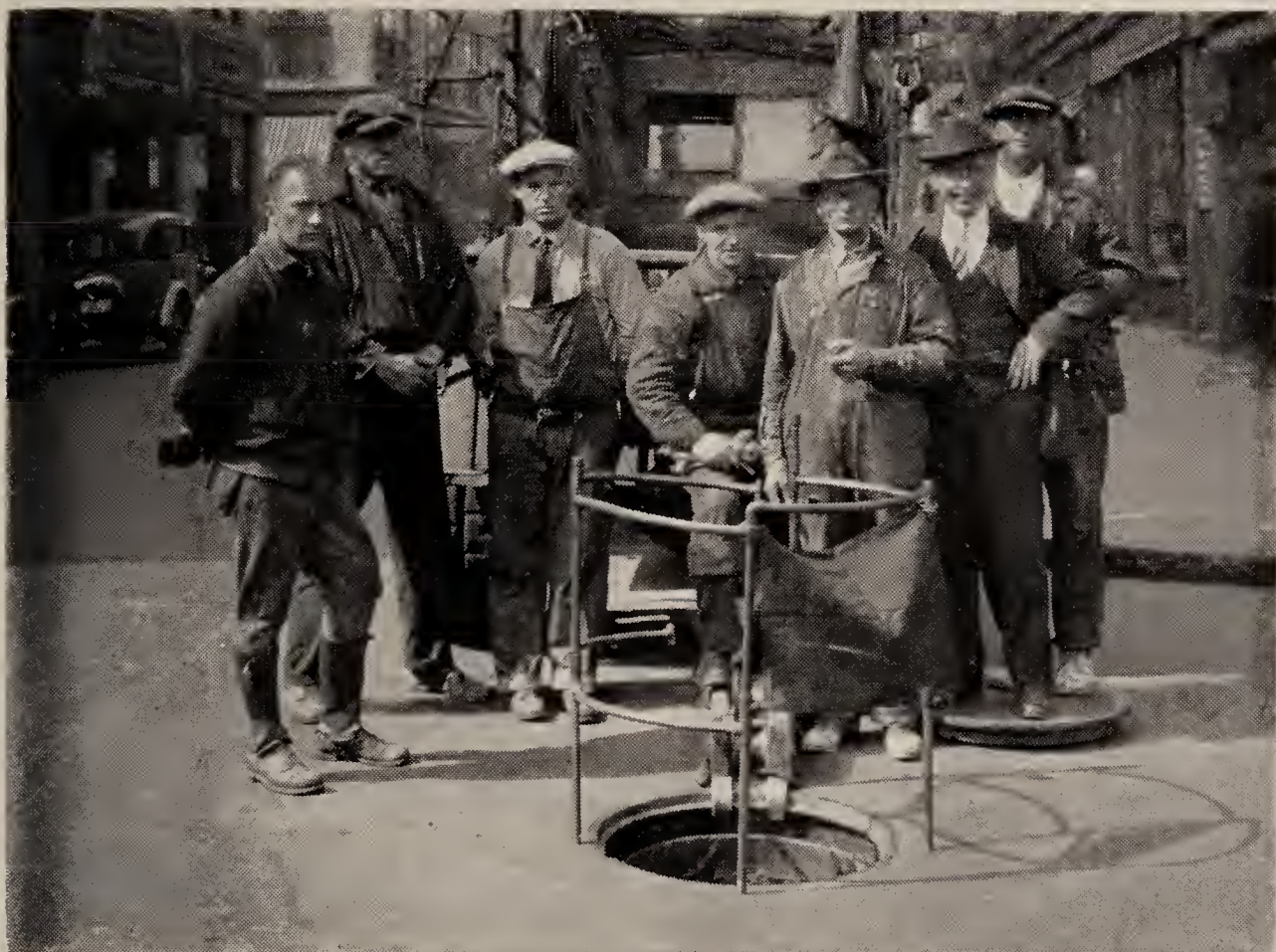
THE GANG THAT PULLED IN THE 1800-PAIR CABLE—1928
